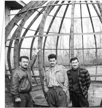
CONSTRUCTION OF LANGAROU DOME IN 1997
